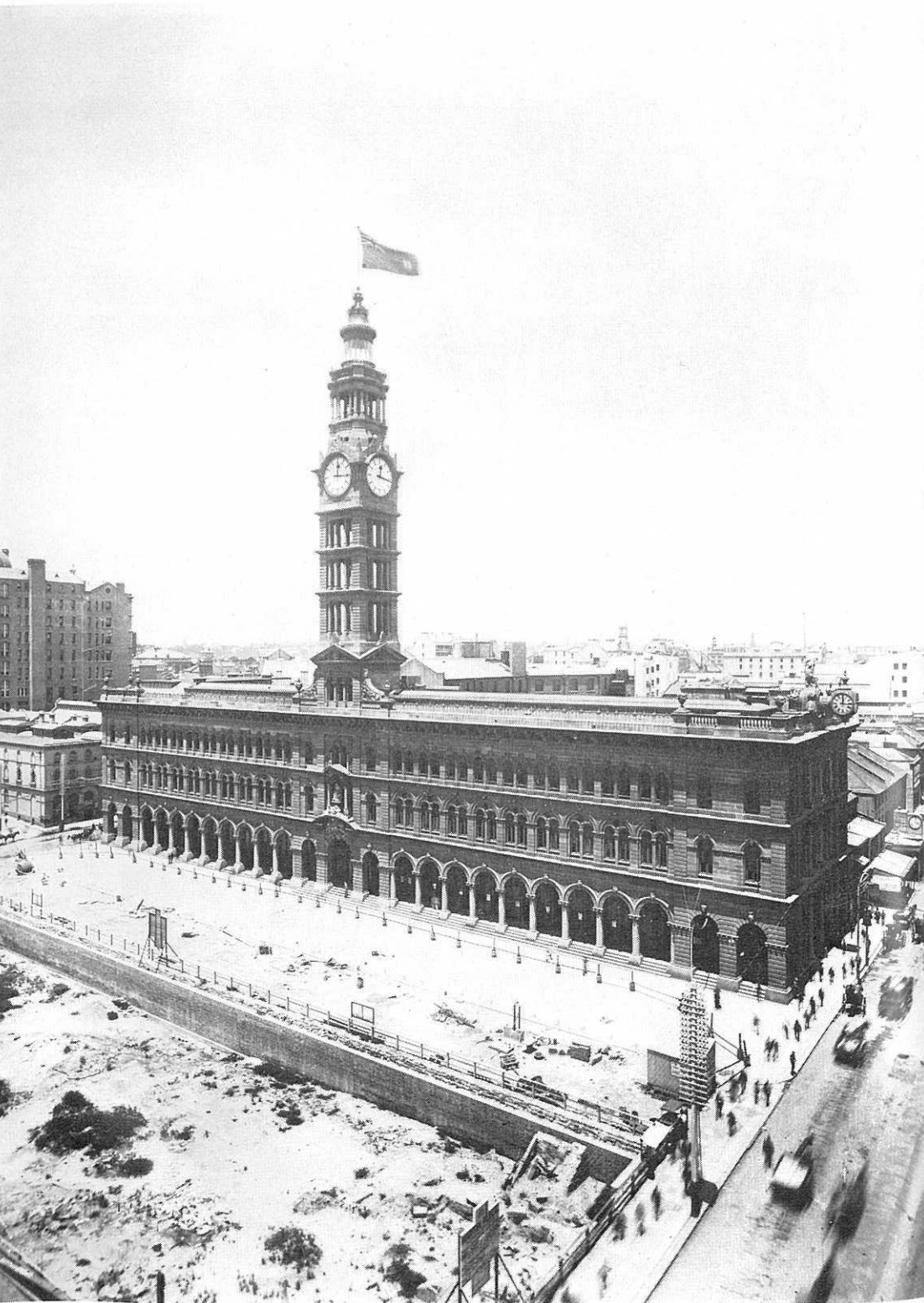
Demolition of buildings to form the new Martin Place (1892)
